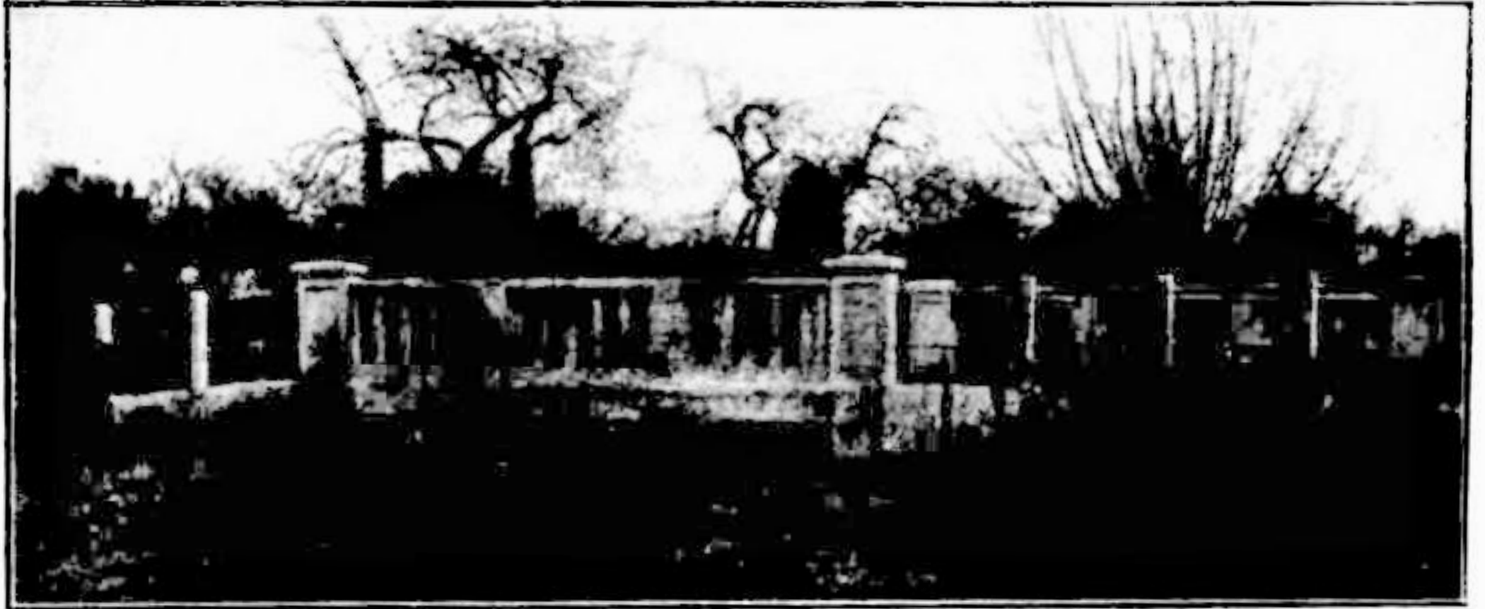
A view of the new bridge.
