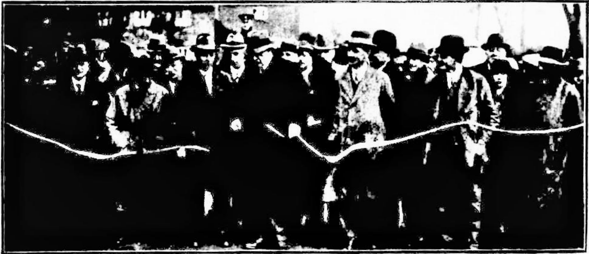
Mr. E. M. Sturges, Chairman of the Wokingham Rural District Council, cutting the tape and opening the bridge.
