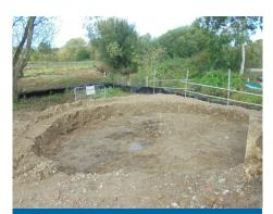
Ground preparaton for caissons which will be used for the foundation of the new footbridges in the Emmbrook watercourse
