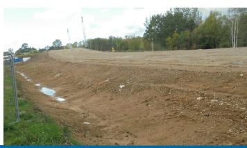
Finished embankment leading to the new railway bridge. The embankment is 8m higher than the original ground. The finished level of the embankment is expected to be at the same level as the M4 as this is the height required to clear the railway
