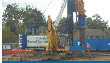
Rotary excavation for the piles is progressing. Piling work is taking place on both sides of the railway simultaneously. The tall blue cranes can be seen from the Reading Road and surrounding area
