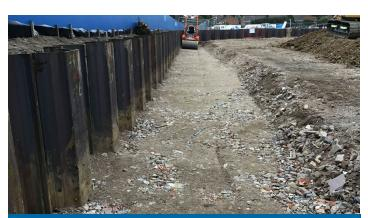
Sheet piling installation completed. The system will protect the railway during the new bridge piling work
