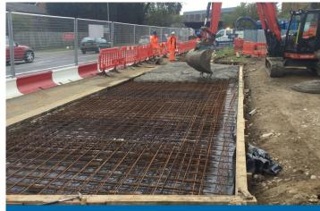
New temporary site access by the BP garage on Reading Road where existing underground utilities are being lowered
