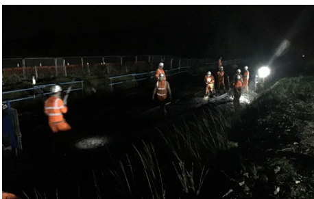
Overnight works which included site clearance, installation of fencing and a track monitoring system were carried out along the railway track.
