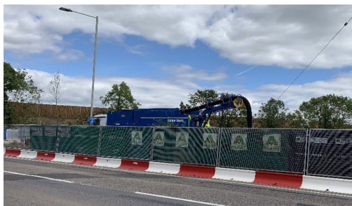
The asset mass barrier on Reading Road is a protective steel barrier consisting of hot galvanised elements powder coated in highly visible safety colours. Individual base units weigh 55kg and each unit links together via vertical pins
