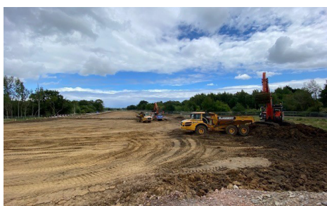
Top-soil strip along a section of the new Distributor Road
