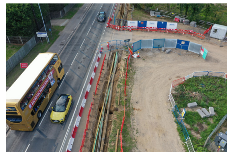
Uncovered utilities on Reading Road
