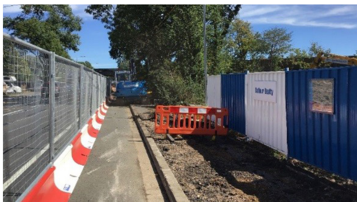
The asset mass barrier on Reading Road is a protective steel barrier consisting of hot galvanised elements powder coated in highly visible safety colours. Individual base units weigh 55kg and each unit links together via vertical pins
