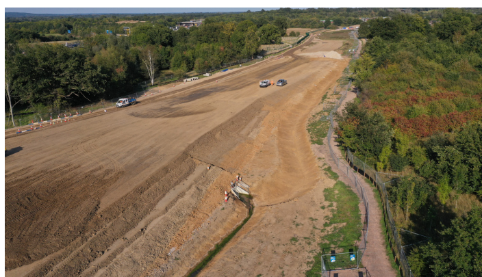
New Distributor Road
