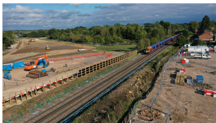
Railway crossing and new Distributor Road
