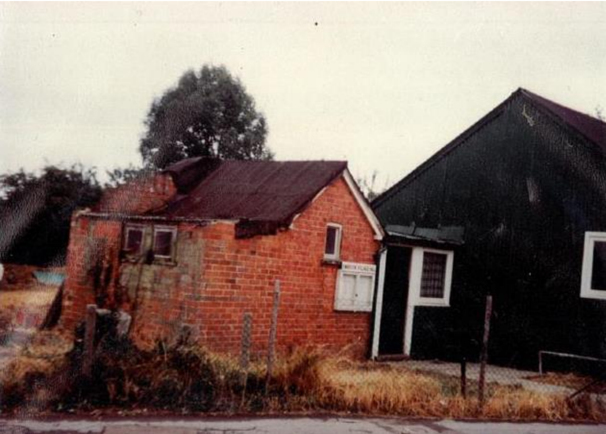
The Old Toilet Block - 1977
