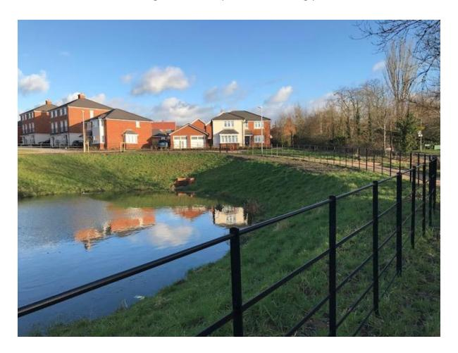
The attenuation pond is now fenced off with a life ring installed to meet the safety standards set by you.
